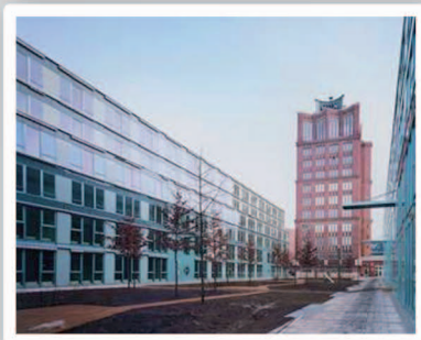
Beton-Sandwichelementen Concrete sandwich elements Bürohaus Herlitz, Berlin
